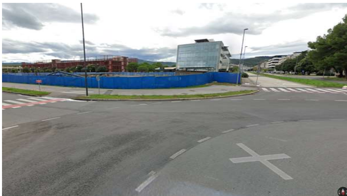
Slika 5: Obstoječe stanje - zaključek kolesarske poti na Ferrarski ulici, (Vir: https://www.google.com/streetview/ )
